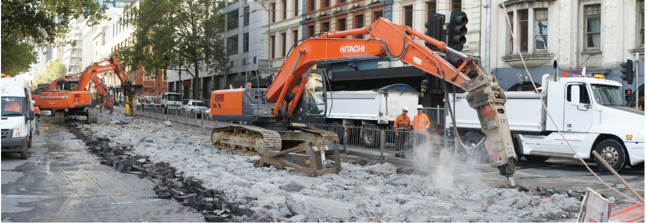
Heavy machinery will be used during the works.
